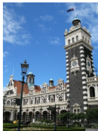
DNN Railway Station C.GTC.NZOTG.02 C.GRC.NZOTG.02
