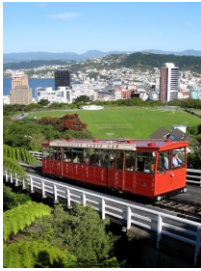
Cable Car C.GTC.WLG.01 C.GRC.WLG.01
